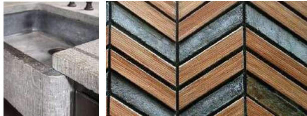
NEW CONCRETE TEXTURED WASH HAND BASIN AND CHEVRON CLAD FRONTAGE WITH INSET TIMBER PLANKS
